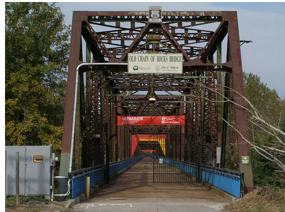
Chain of Rocks Bridge
